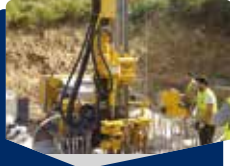
Concrete piles coring
