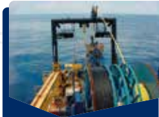
Pipeline lay support and touchdown monitoring
